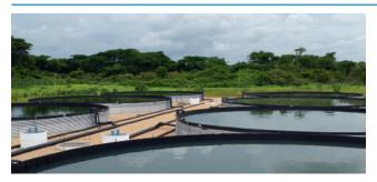
Fish farms use tanks for breeding fish in different stadia. Tilapia, trout, eel, salmon and carps are the most popular for fish production. Installation of fish tanks demands local limited installation knowledge, material and equipment. Steel tanks for fish production are in general supplied in height 1,59 meter. Specific solutions for cleaning and emptying these tanks is a part of our concept.
