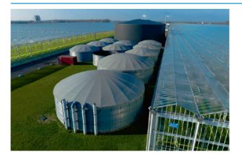
The BUWAdome is a completely covering lightweight frame roof system available for water tanks till a diameter of 15 meter. The system consists of an aluminium tube frame that dispenses its own weight onto the water tank. The cover material is a reinforced PVC quality and is installed on the frame afterwards. The cover is produced with a manhole so you can get in the water tank.
