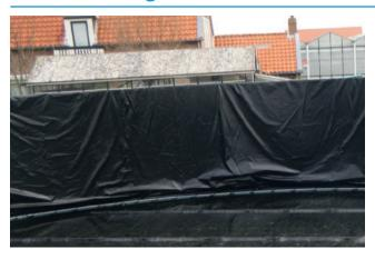
This cover is floating on the water surface. This floating cover has a reinforced hem with rings for fastening. For floating capacity, a rack of PVC pipes should be constructed (Ø 63 mm), which has to be obtained from a local supplier. The cover must be stretched around this rack. The system protect the water against algae growth, but reduce also evaporation and waves inside the tank. This cover fits for water tanks with a minimum diameter of 8,5 meter.
